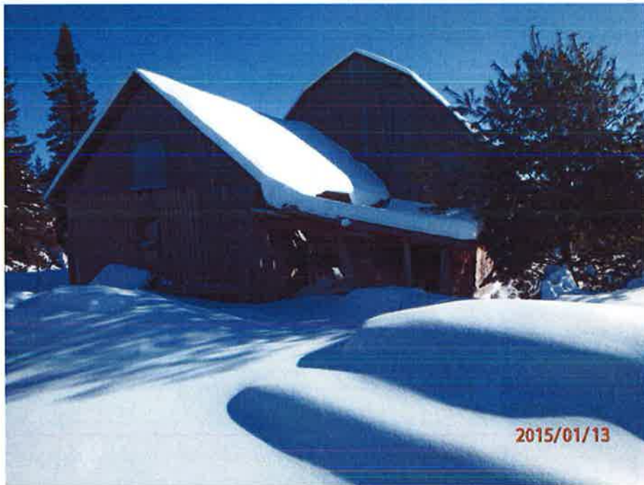
Shed located on the northwest corner of the barn.
