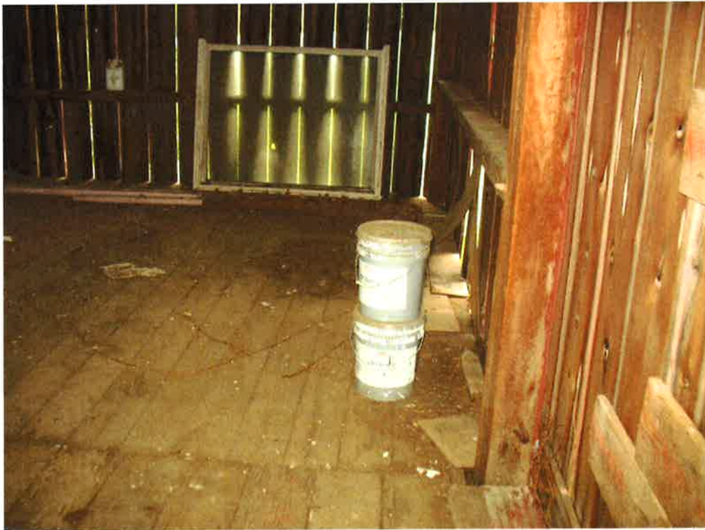
Photo 12 - View of paint pails, upper level of barn, west wall.
