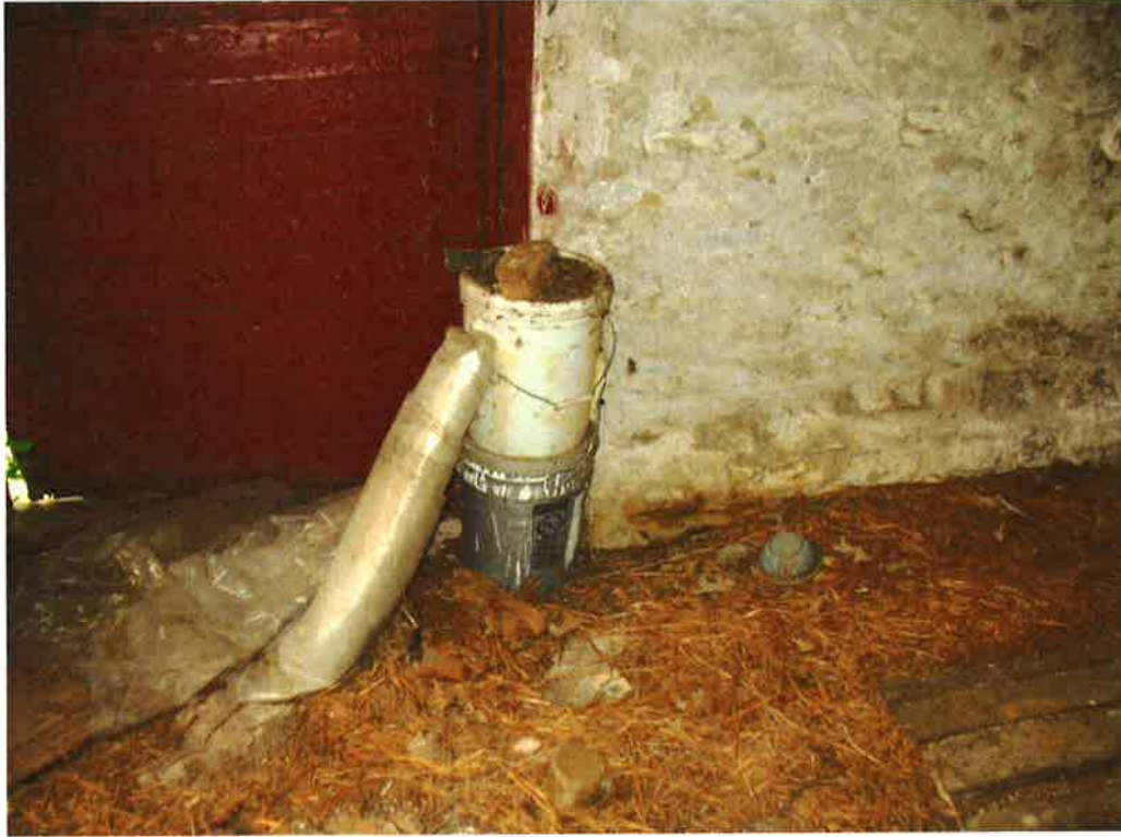
Photo 11 - Paint pails, lower level of barn, northeast corner.
